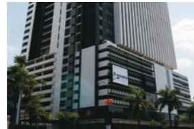
Malaysia Plaza 33 Office Block A
