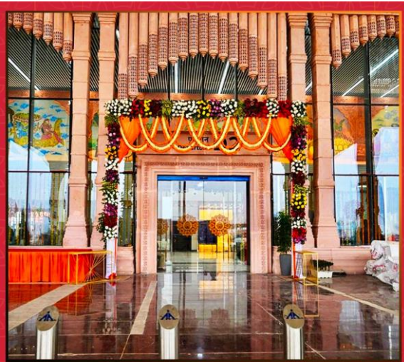
Hitachi Cooling & Heating: VRF Iconic Site Project :Maharishi Valmiki International Airport Ayodhya Dham
